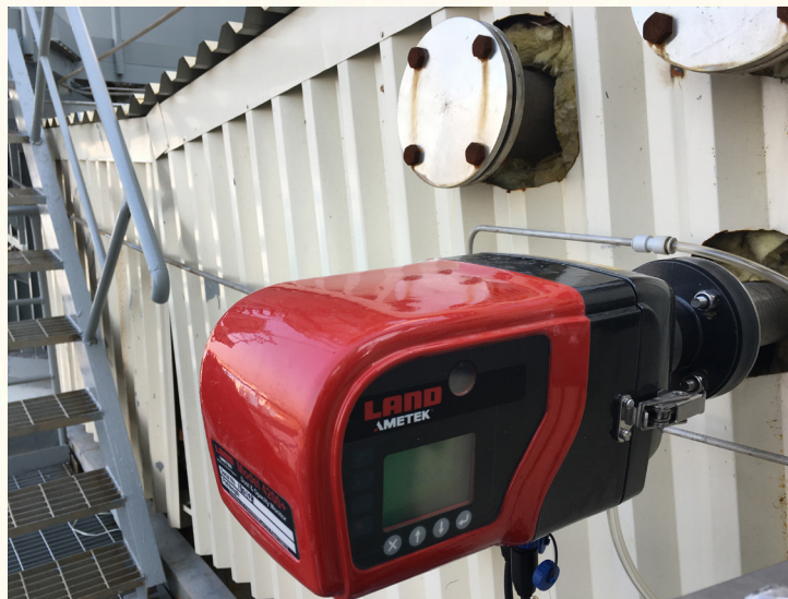
Figure 1. AMETEK Land 4500 MkIII transceiver installed on a power plant duct.
